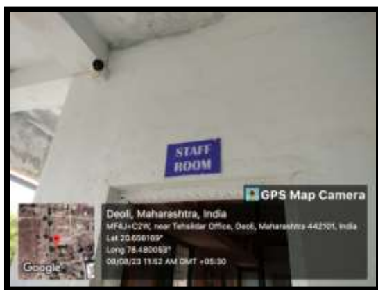
CCTV camera in staffroom
